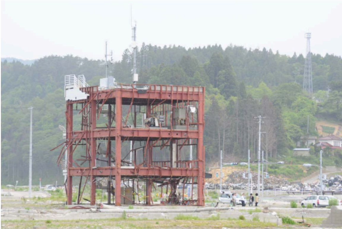
Figure 2: Destruction from the Great East Japan Earthquake
